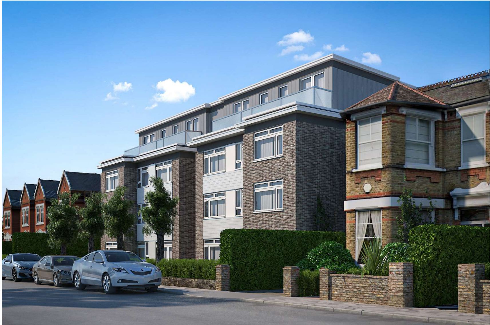
CGI View along Prince's Road looking East
