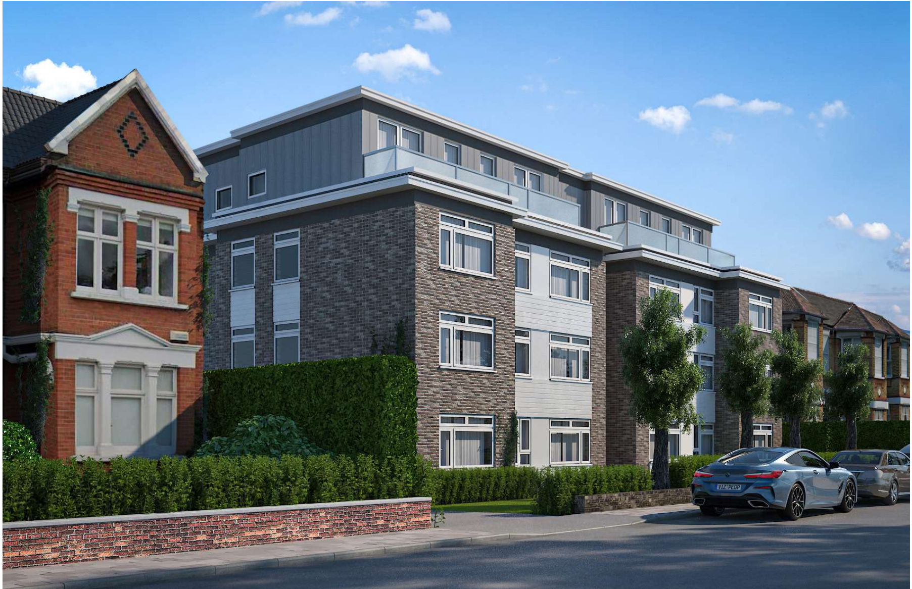
CGI View along Prince's Road looking West
